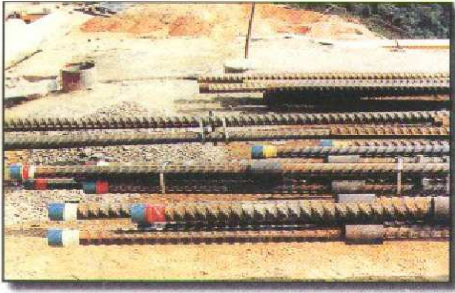
Micro piles & Soil Nails
