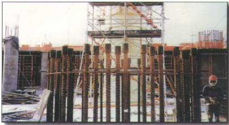
Columns and Piles
